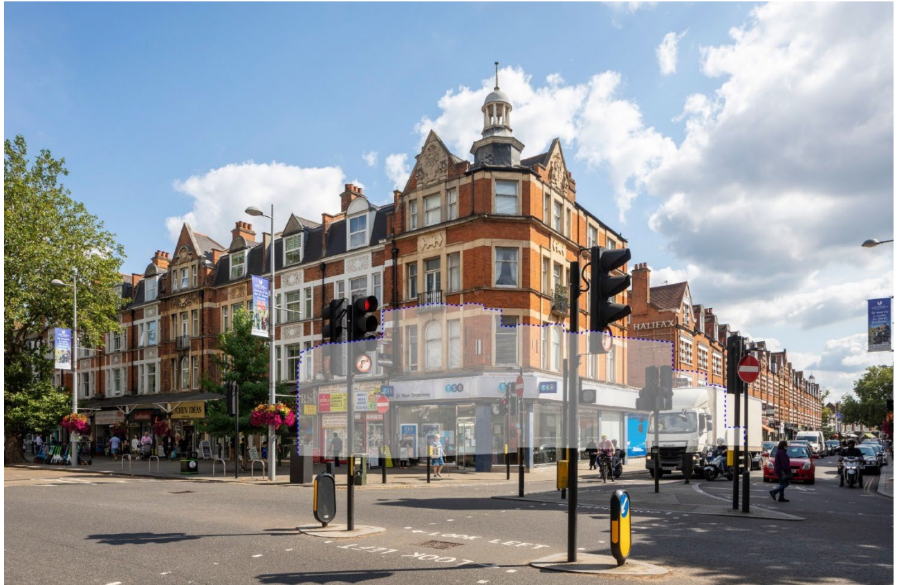
Figure 26: View of proposed development at the New Broadway and Bond Street junction
